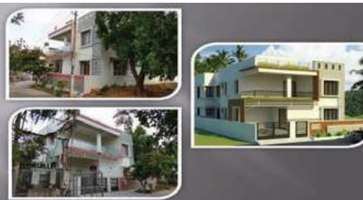
Project Location:- Sarjapura Road, Bangalore Project Description:- The structure was designed for G+2+Terrace Floors only & executed for G+1+Terrace Project size & scale:- 40'x70' & 84,52,000.
