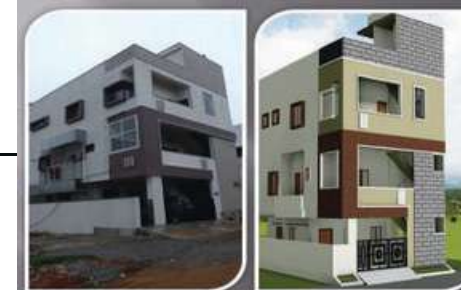
Project Location:- Kudlu Gate, Bangalore Project Description:- The structure was designed for G+1+Terrace Floors Project size & scale:- 30'x40' & 60,00,000
