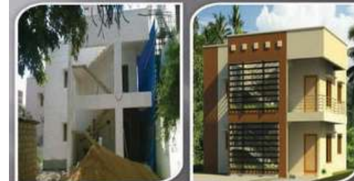
Project Location:- Banaswadi, Bangalore Project Description:- The structure was designed & executed for G+1+Terrace Floors only. Project size & scale:- 40'x30' & 38,24,000
