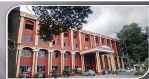
Project Location:- Tumkur Project Description:- Renovation work for court building Tumkur.
