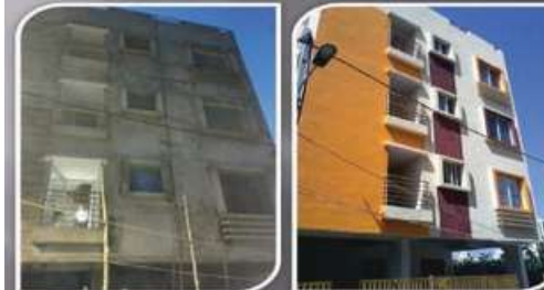
Project Location:- HSR Layout, Bangalore Project Description:- The structure was designed & monitored for G+3+ Terrace Floors only. Project size & scale:- 40'x50' & 67,20,000
